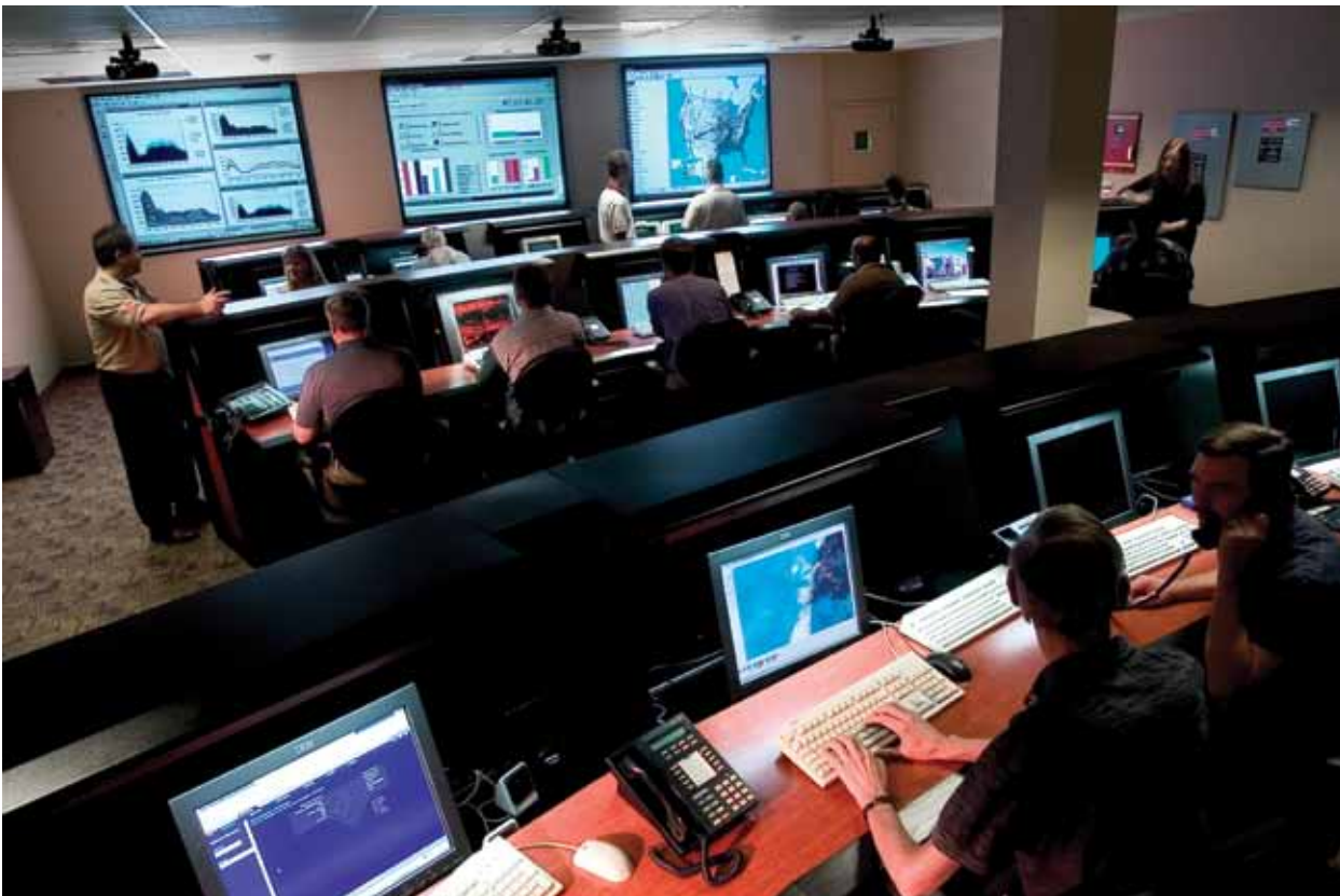
The global IT control room in Chandler, Arizona, is the heart of our communications, data storage and business activities with customers and suppliers.
